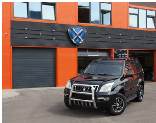
ALUTECH sectional doors installed in a car wash
