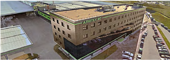
Alutech Doors Systems, LLC
